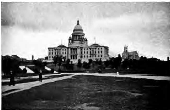
The Rhode Island State House at Providence
